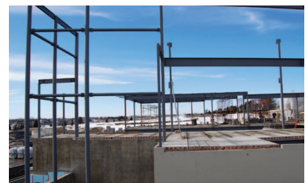
View of east entrance
